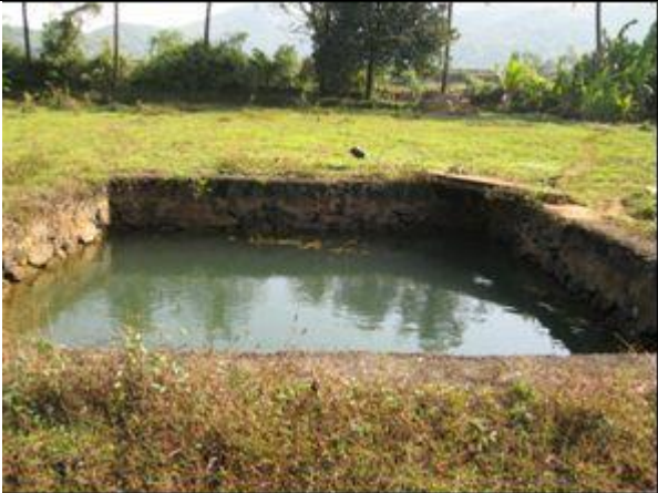
Photo 18: Ground water level in the open dug well at the toe part of the slide
