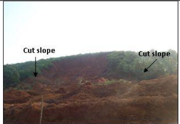
Photo 6: View of the landslide from the toe of the slide showing the original cut slopes
