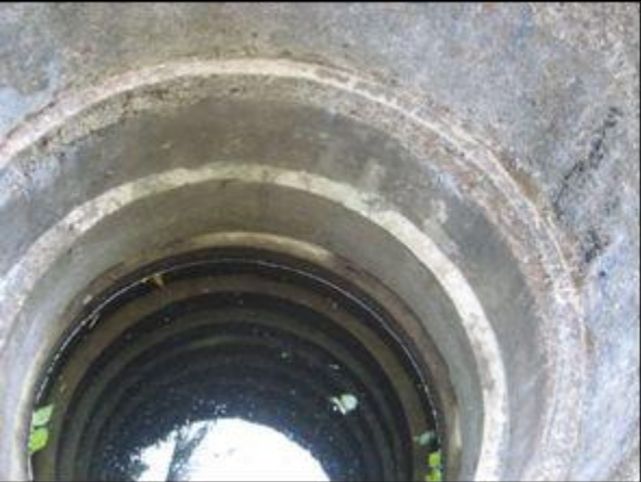
Photo 17: Dug well at the toe
