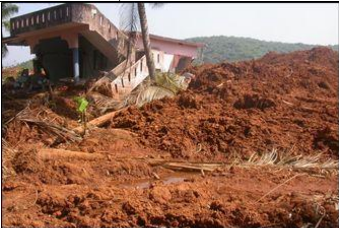
Photo 9: The damaged house that has been carried down slope by about 15 m, near the toe part of the Kadwad land slide
