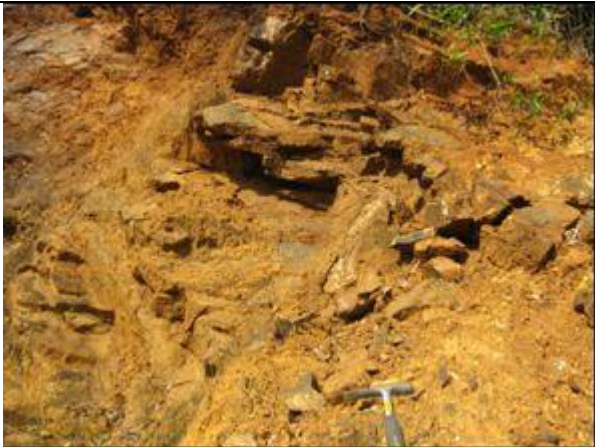
Photo 16: Weathered granite (saprolite) in the slide debris in the mid slope (left flank)
